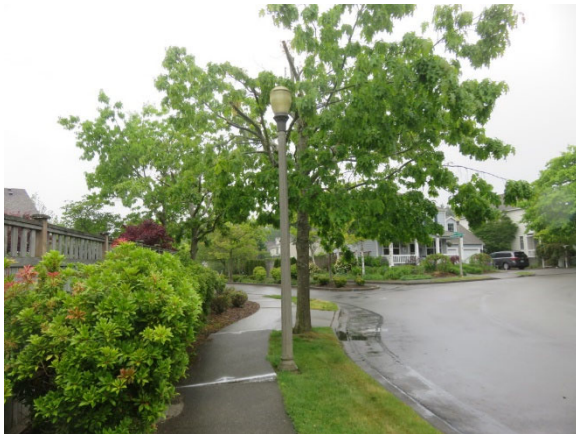
Typical Concrete Light
