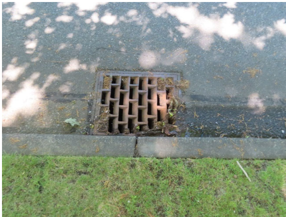
Typical Storm Drain
